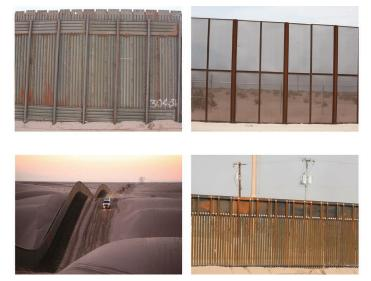
This shows variations in materials used to construct the International Border Fence to accommodate for changes in topography and climate. (Top Left - Landing Mat; Top Right - Secondary; Bottom Left -Floating; Bottom Right - Bollard)
