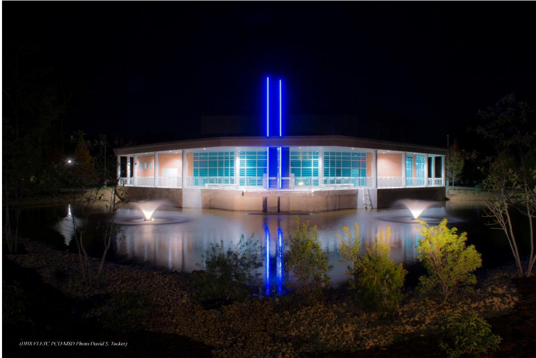
Back Deck of FLETC-Glynco Building 912
