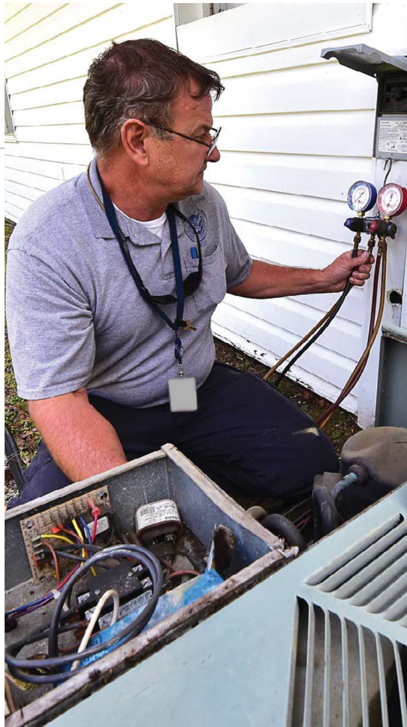
James Winslett performs maintenance on an air conditioning unit. (Photo by David Tucker, FLETC)
