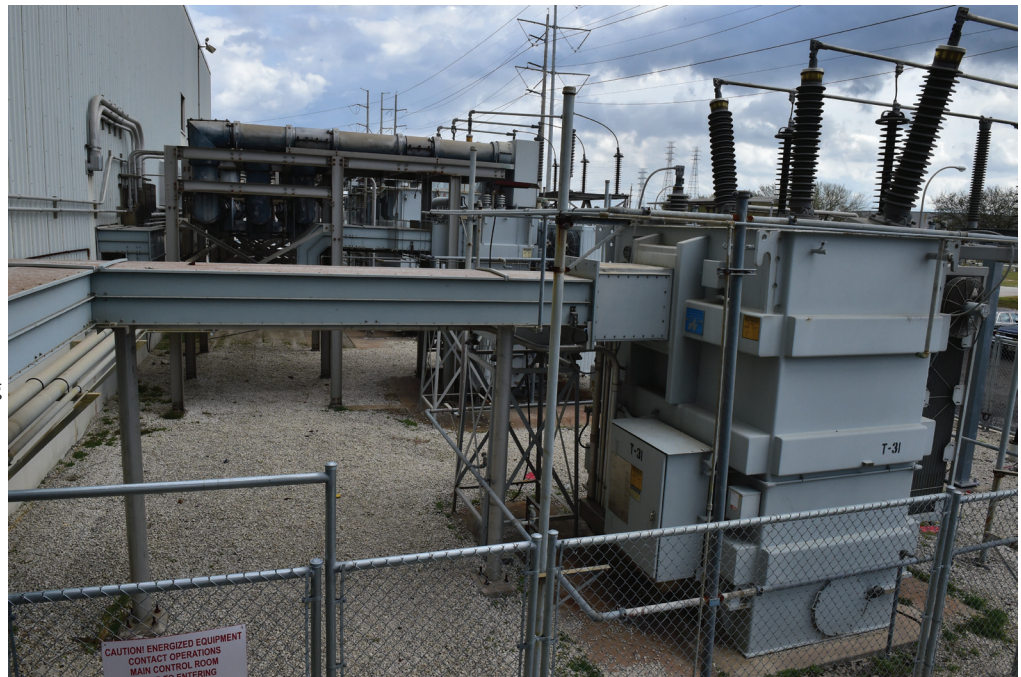
LEFT: An advanced student in the Federal Law Enforcement Training Centers (FLETC) Critical Infrastructure Security and Resilience Training Program assesses a major electricity generation plant. RIGHT: The plant provides 1,300 megawatts during peak capacity and can provide electricity for over 250,000 households.
