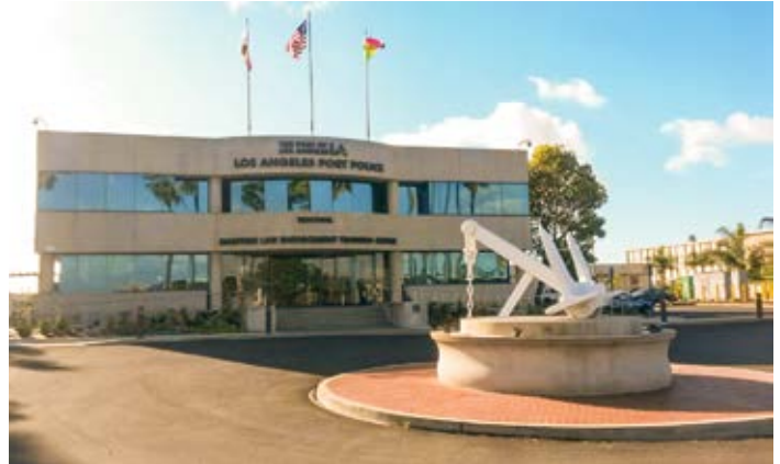
The Los Angeles Regional Maritime Law Enforcement Training Center Front Entrance.
