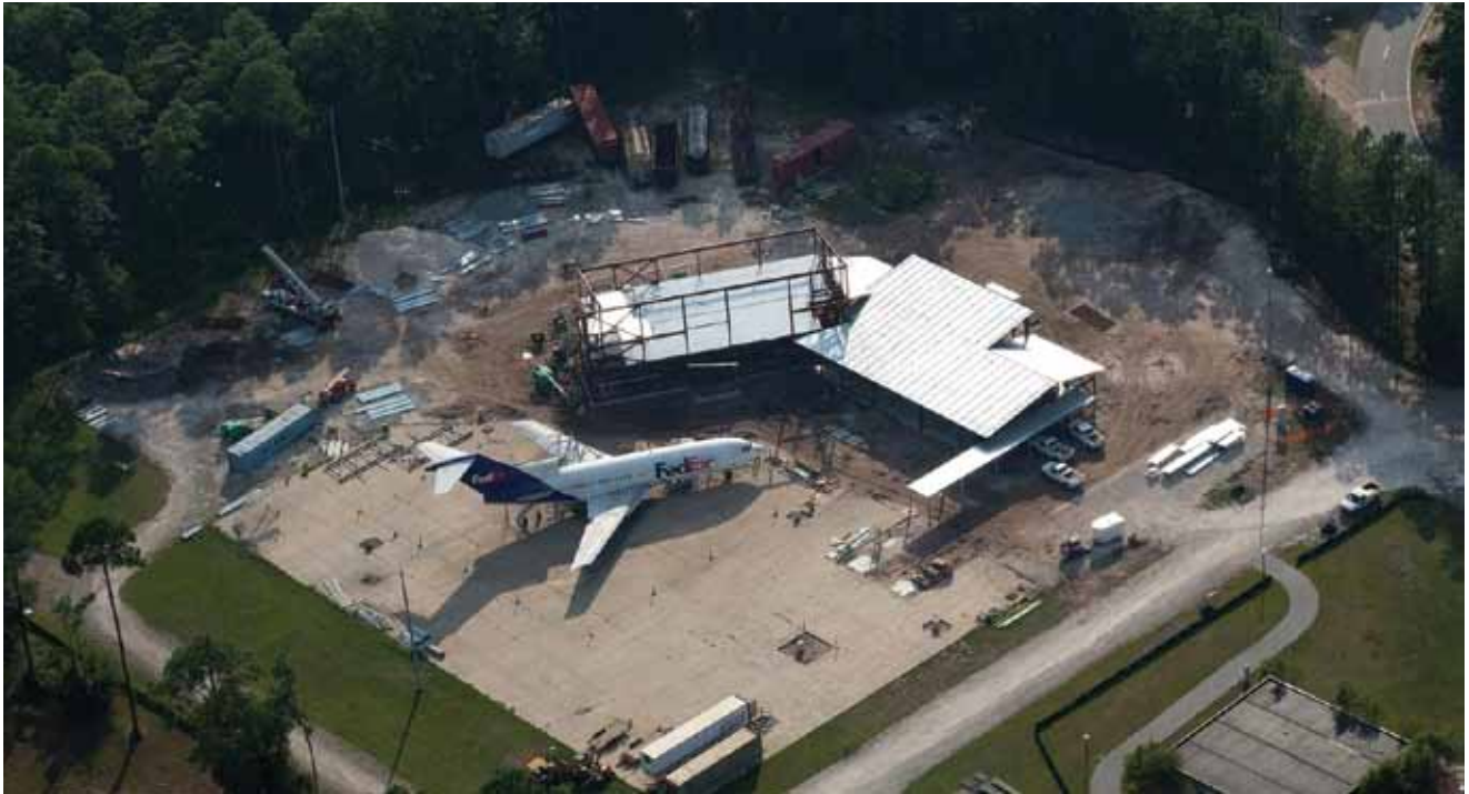
17 The new FLETC Intermodal Training Facility under construction
